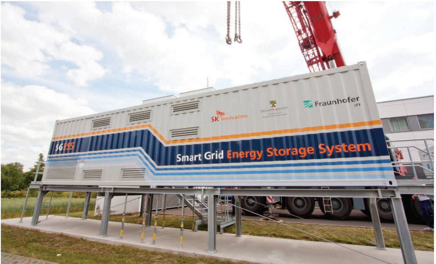
The Fraunhofer IFF's mobile energy storage system. Five thousand battery cells are in the container. (See the photo on page 26). Photos: Fraunhofer IFF, Daniela Martin
