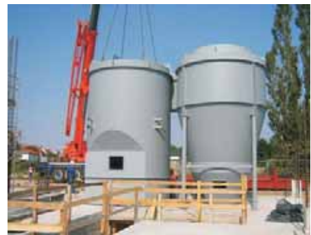
Fig 2: Steelwork for the firing plant. Photo: Matthias Gohla
