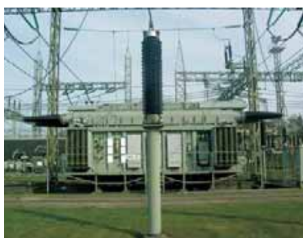
Fig. 1: A 200 MVA mobile network transformer in RWE Netzservice's Niederrhein switching station and as a VR graphic on the right. Photo: Wilhelm Termath
