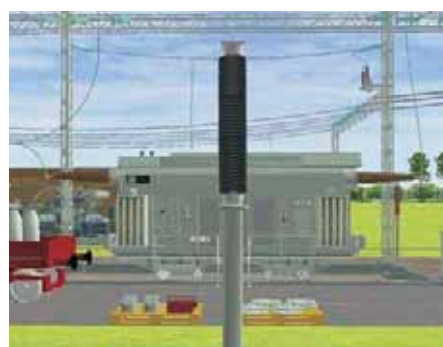
Fig. 1: A 200 MVA mobile network transformer in RWE Netzservice's Niederrhein switching station and as a VR graphic on the right. Photo: Wilhelm Termath
