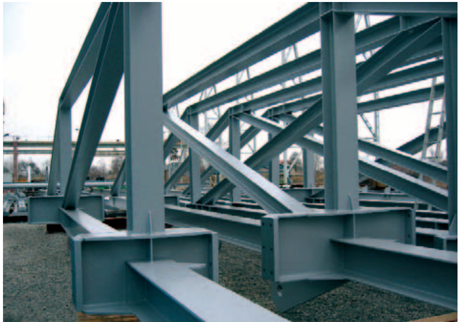
Figure 1: Structural steel elements at a construction site.
